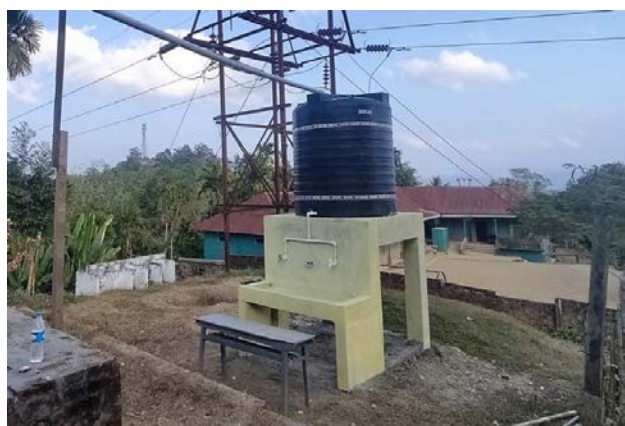
Govt. T. Robert HS (Rain Water Harvesting)
