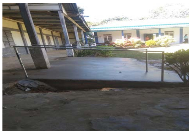
Govt. Kawnpui HS (Ramp with Handrail)
